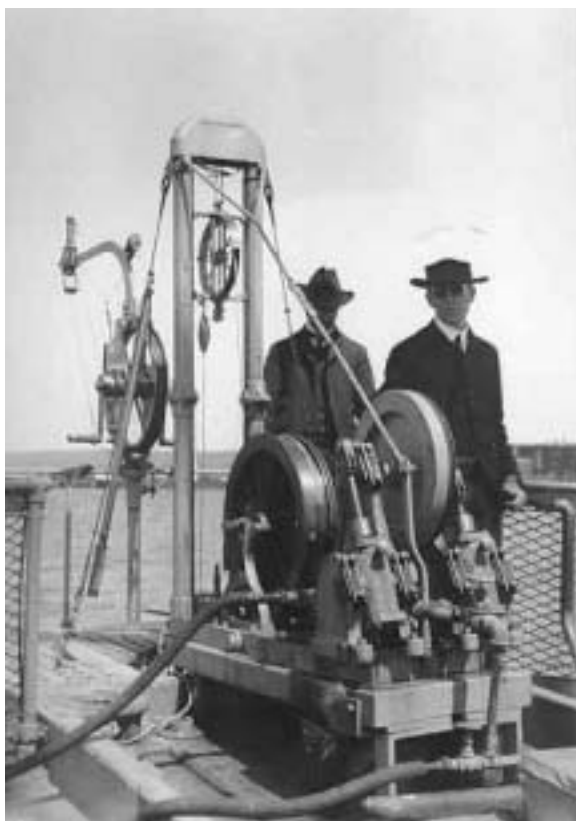
Figure 3. Sigsbee Sounding Machine, R/V Albatross, March, 1904.
